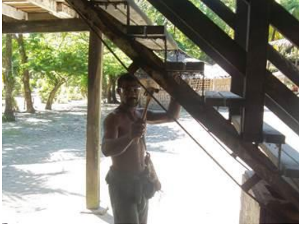
Morea breaking off the chunks of rust
