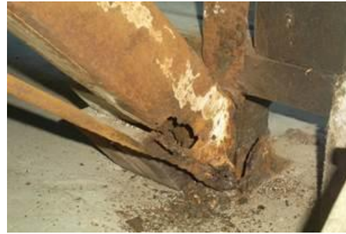
Bottom of the stairs shored up with wood
